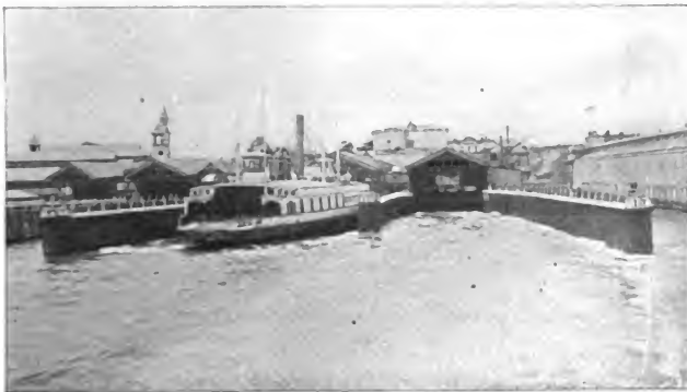
DELAWARE, LACKAWANNA & WESTERN RAILROAD: DEPOT IN HOBOKEN.
